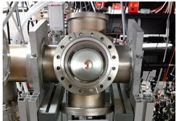
Figure 9: High vacuum tubing when six-way cross was installed with the source removed.
